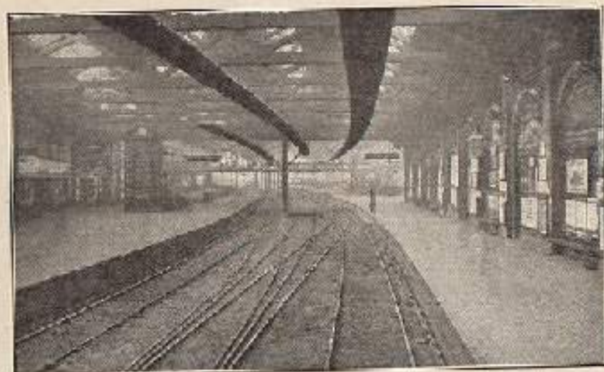
The Main Line Departure Platform at Waterloo.
