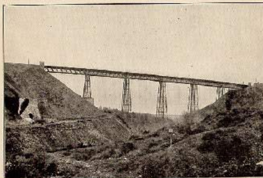
Meldon Viaduct—from the valley.
